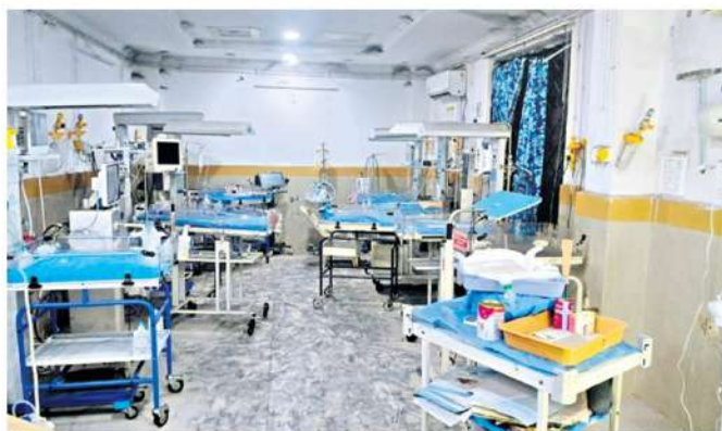
A view of SNCU where the incident occurred at RIMS in Adilabad Monday midnight.
